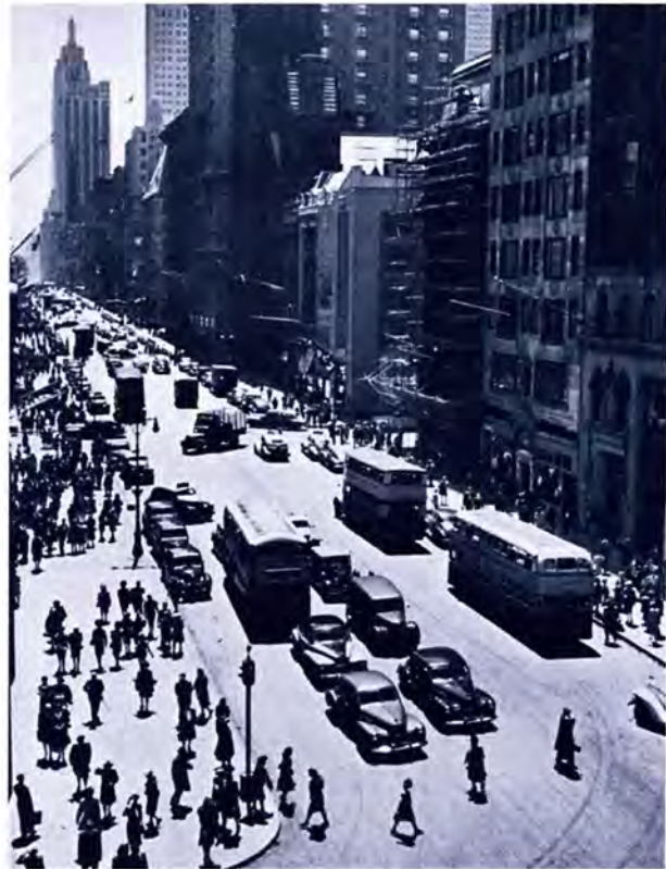
View of 34th Street and Empire State Building, 1940s
