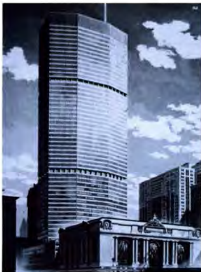
PanAm Building (now Met Life), in which Ernst Stiefel had his office
